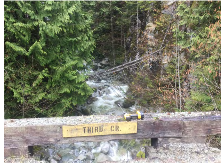
Looking upstream from deck
