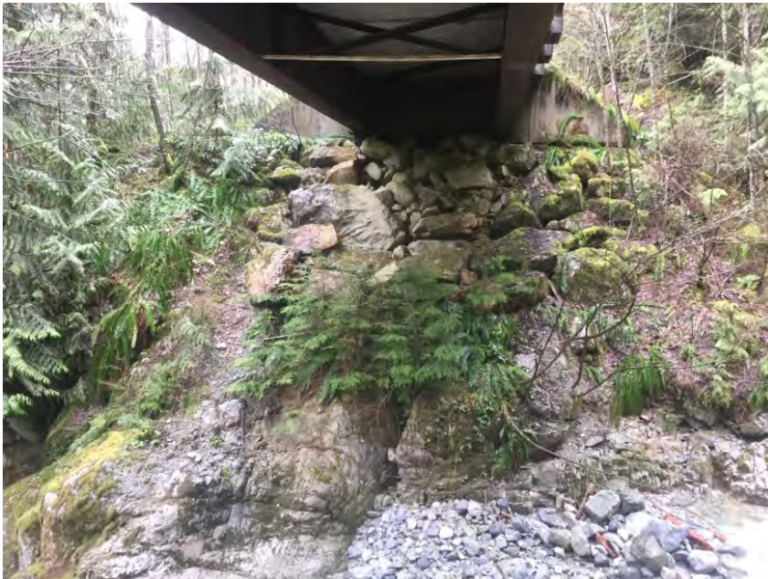
Right Bank Abutment when facing downstream
