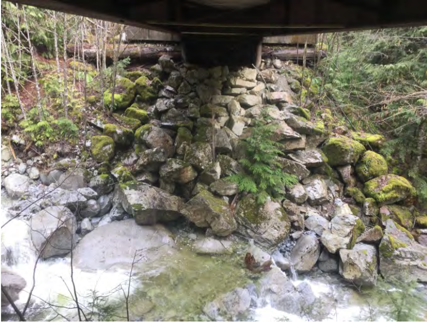
Left Bank Abutment when facing downstream
